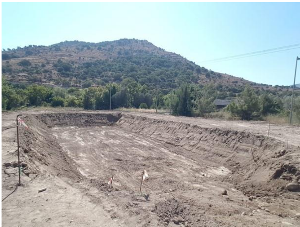
Figure 4.1. Excavation of wetland basins
