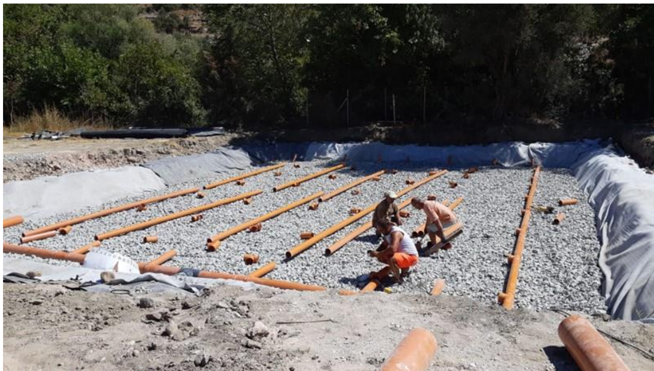
Figure 4.8. preparation of the distribution system in VF SAT
