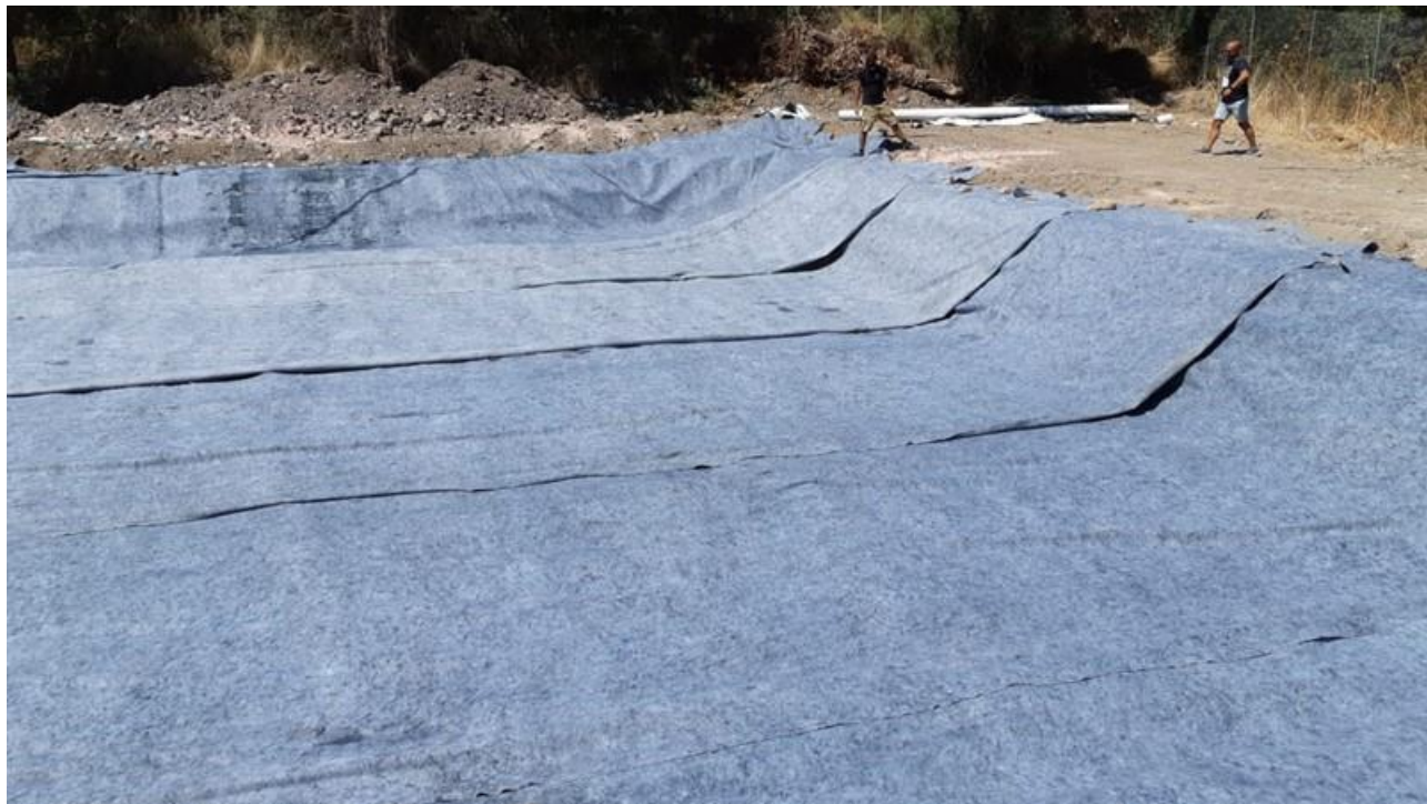
Figure 4.6. placing of geotextile 2nd layer in wetland basins
