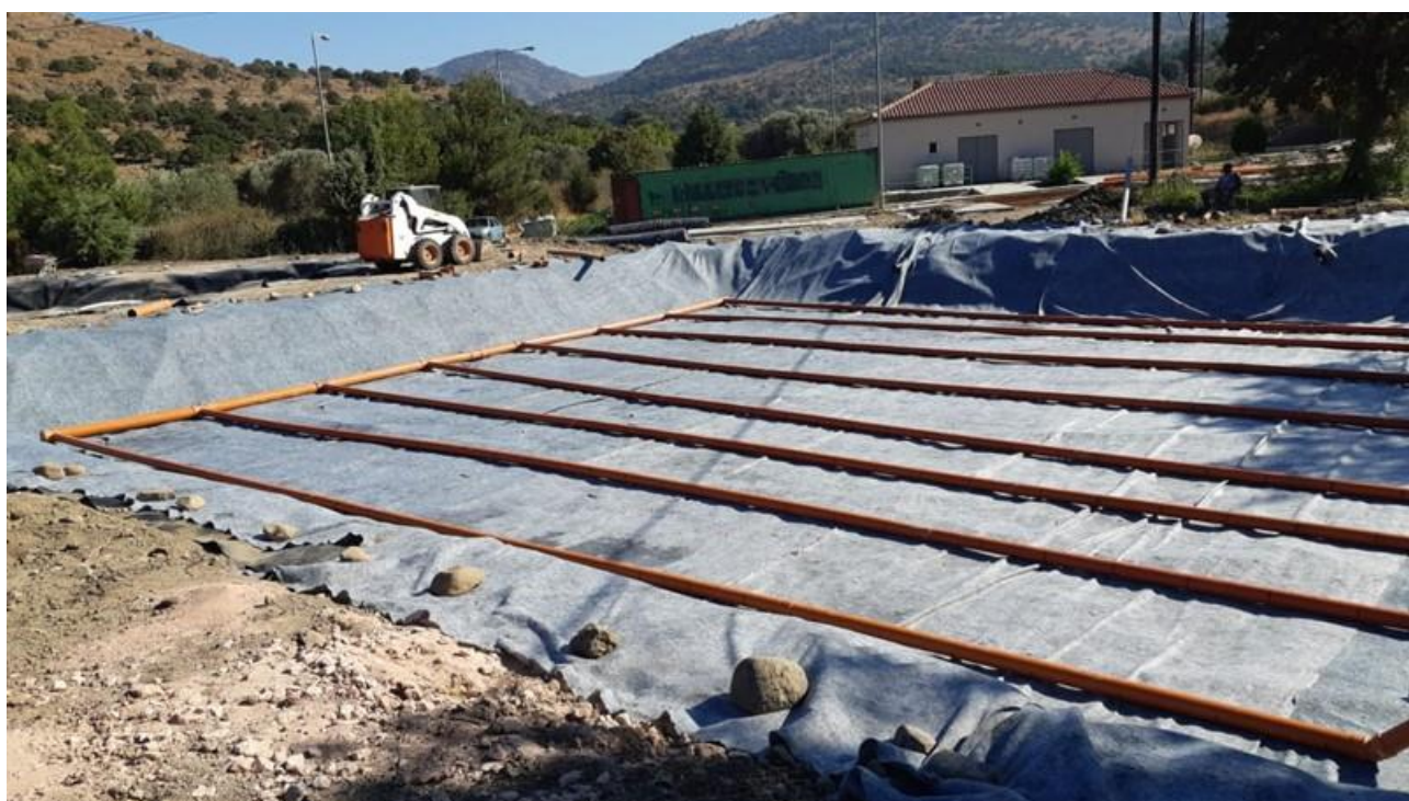
Figure 4.7. placing of drainage system in wetland basins
