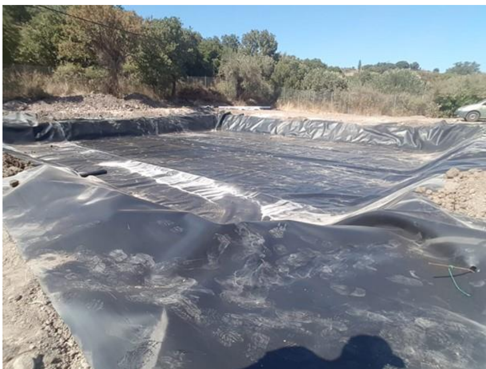
Figure 4.5. waterproofing of wetland basins by HDPE liner
