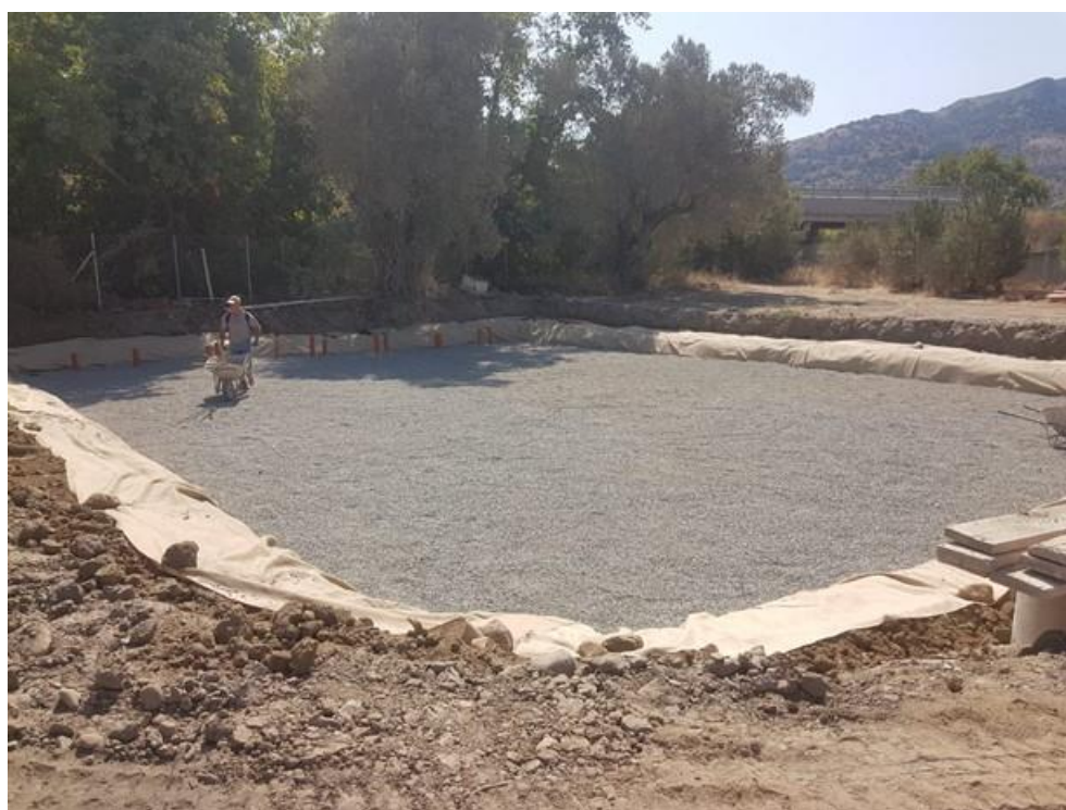
Figure 4.9. placing of gravel and sand material in wetland basins
