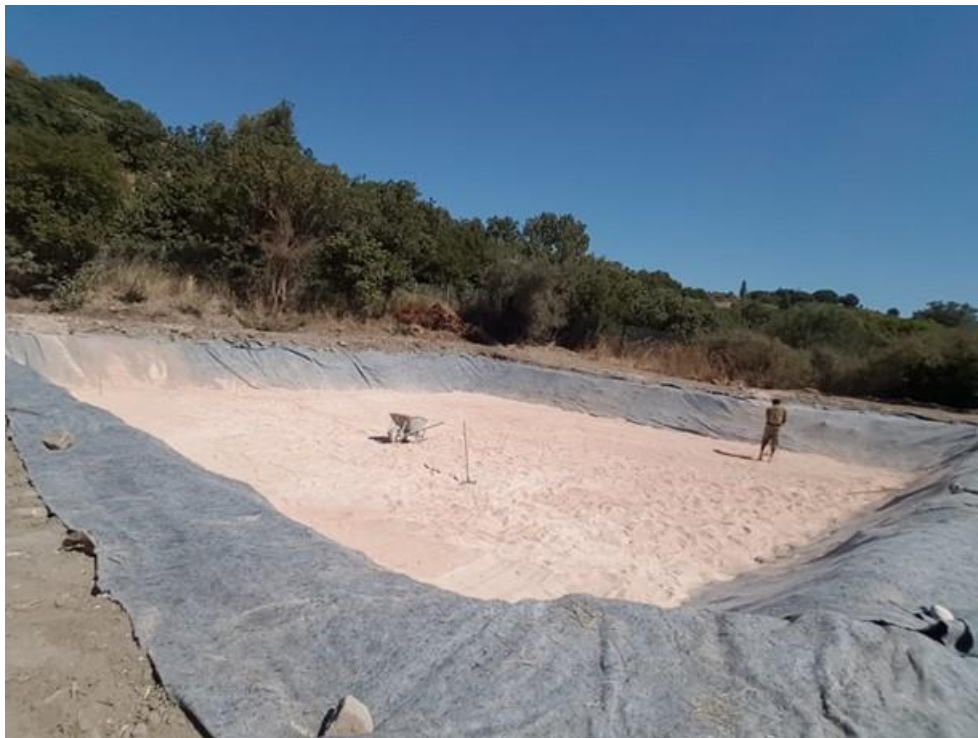
Figure 4.4. preparation of the sand bottom of wetland basins after placing of geotextile
