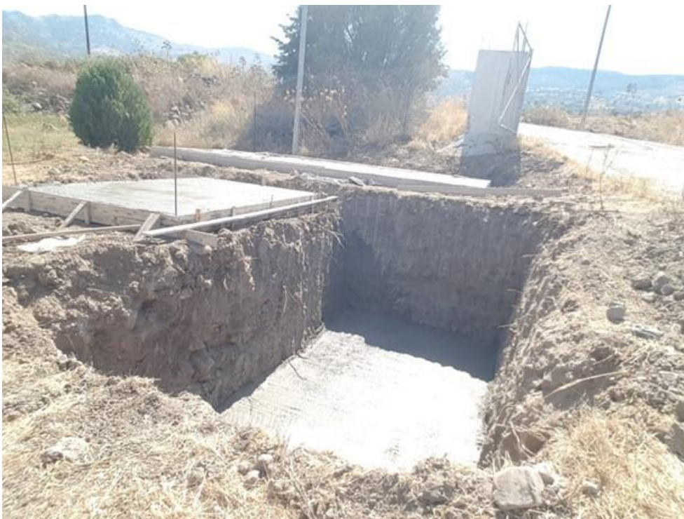
Figure 4.2. excavation for pumping station
