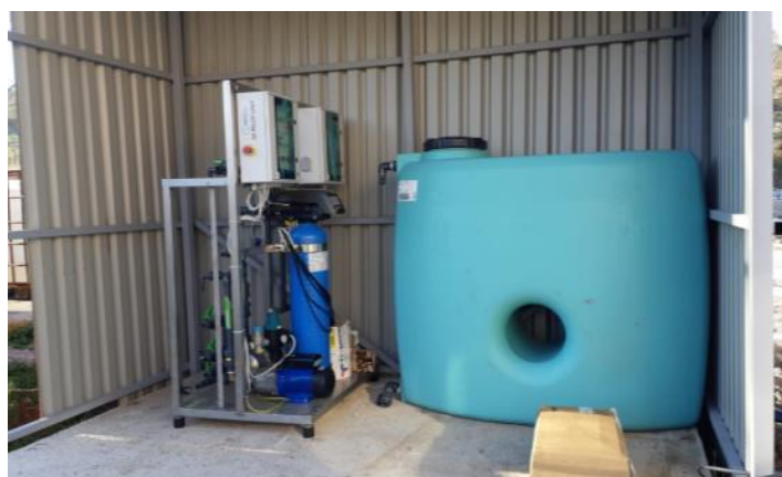
Figure 4.23. Pilot post-treatment unit installed on-site
