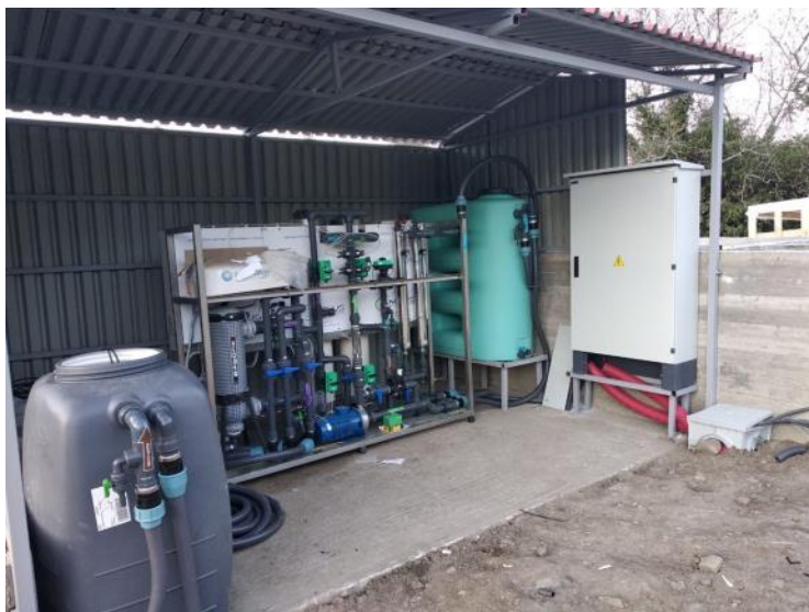
Figure 4.22. Full-scale post-treatment unit installed on-site
