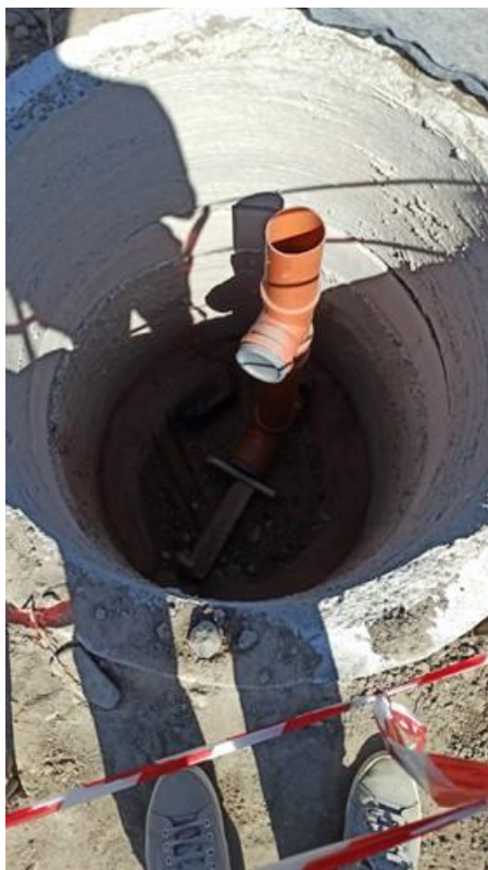
Figure 4.12. water level regulation device for wetland basins
