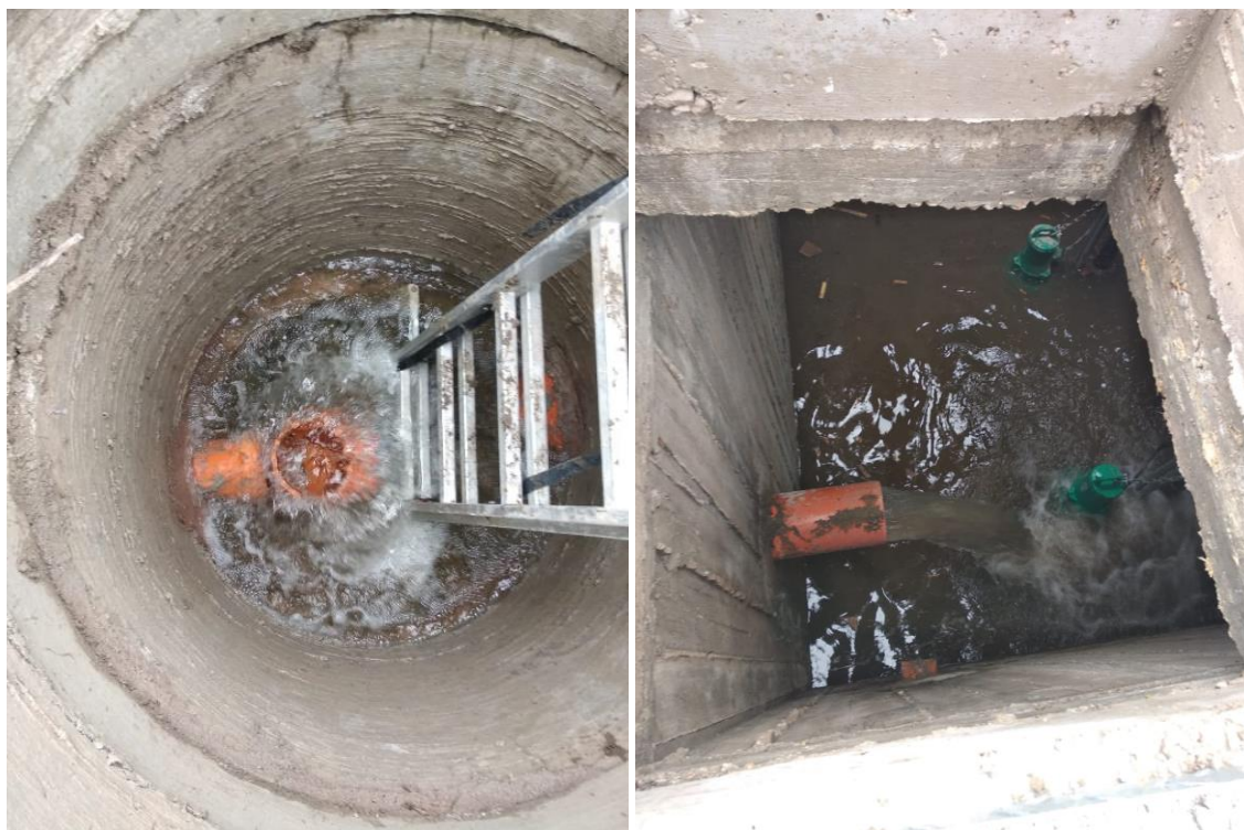
Figure 4.26. SAT CW effluent pit (left) and UNSAT CWs pumping station with SAT effluent (right)
