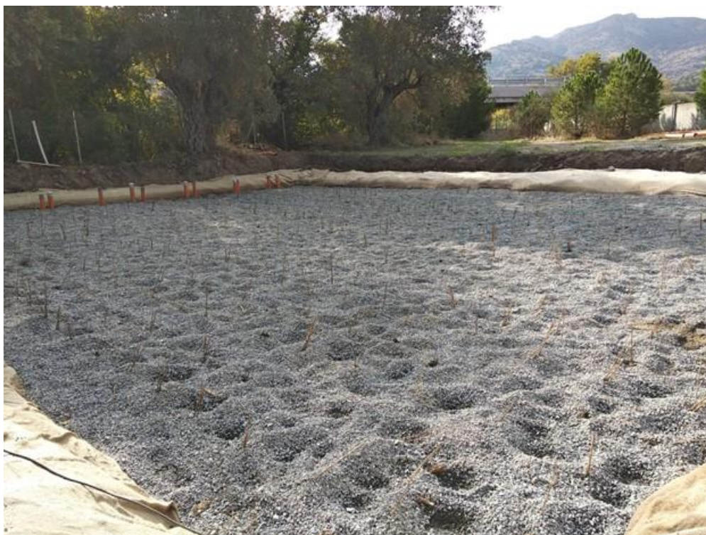
Figure 4.11. placing of plants in VF SAT wetland basin
