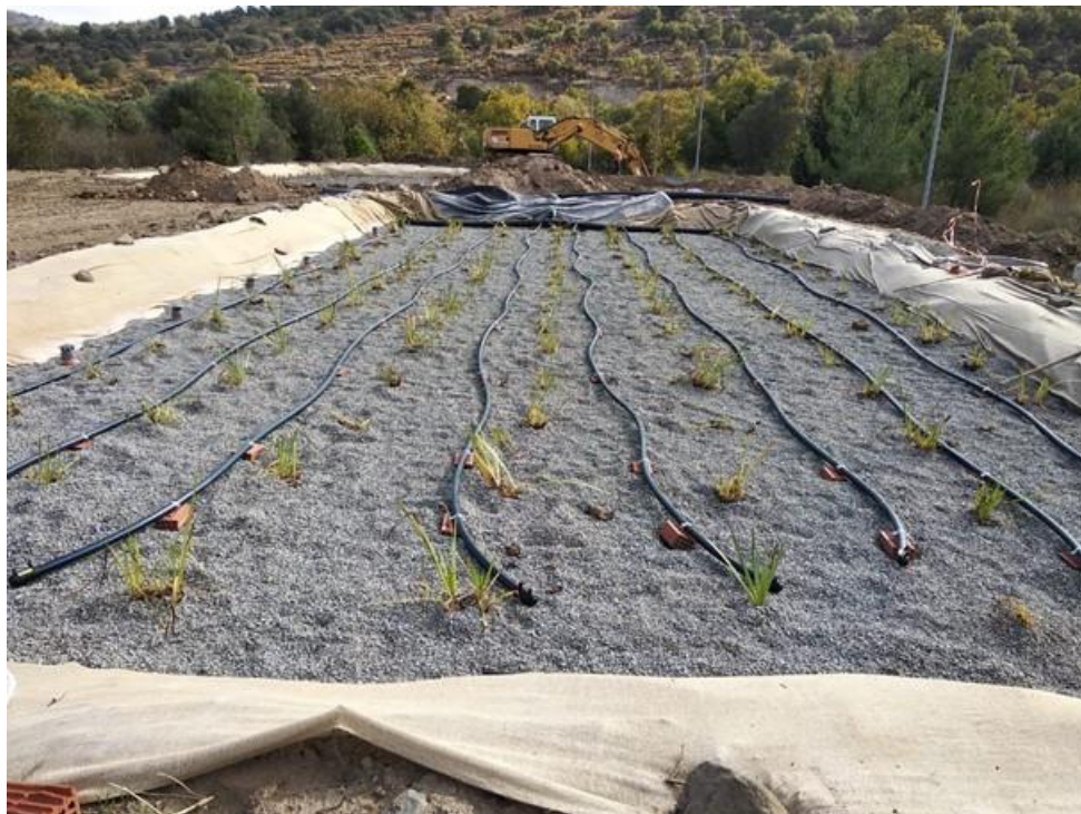
Figure 4.10. placing of plants in VF UNSAT wetland basins
