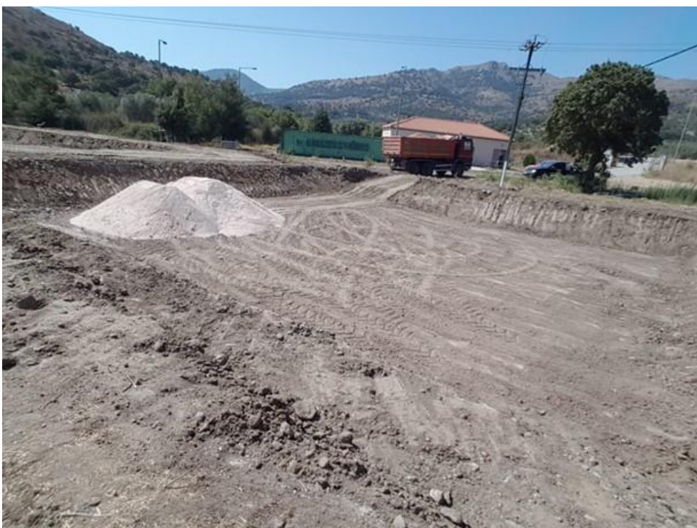
Figure 4.3. preparation of the bottom of wetland basins
