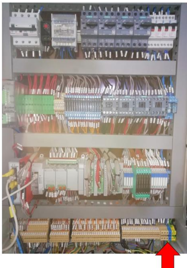
Figure 4.27. Full-scale power supply panel
